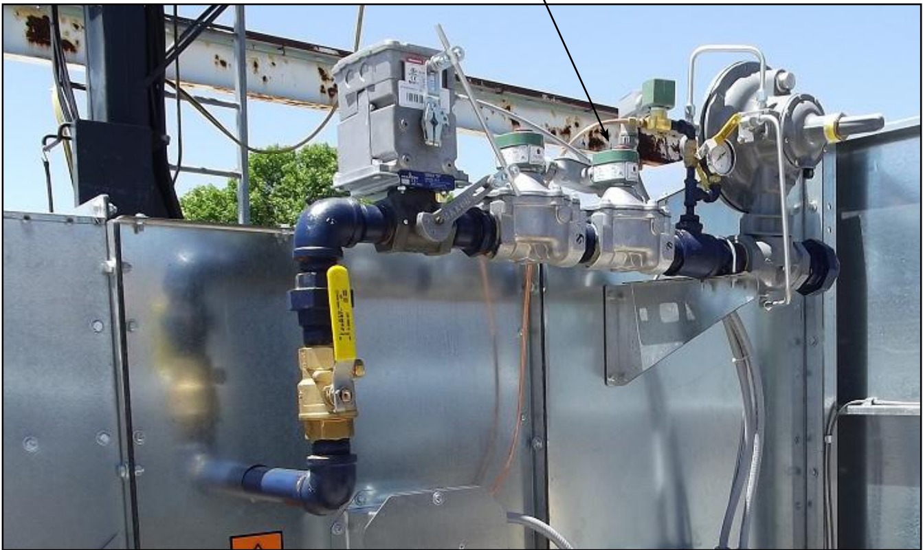
Figure 3.10 - NG Fuel Control Manifold - Dual Solenoid for CE requirements.
