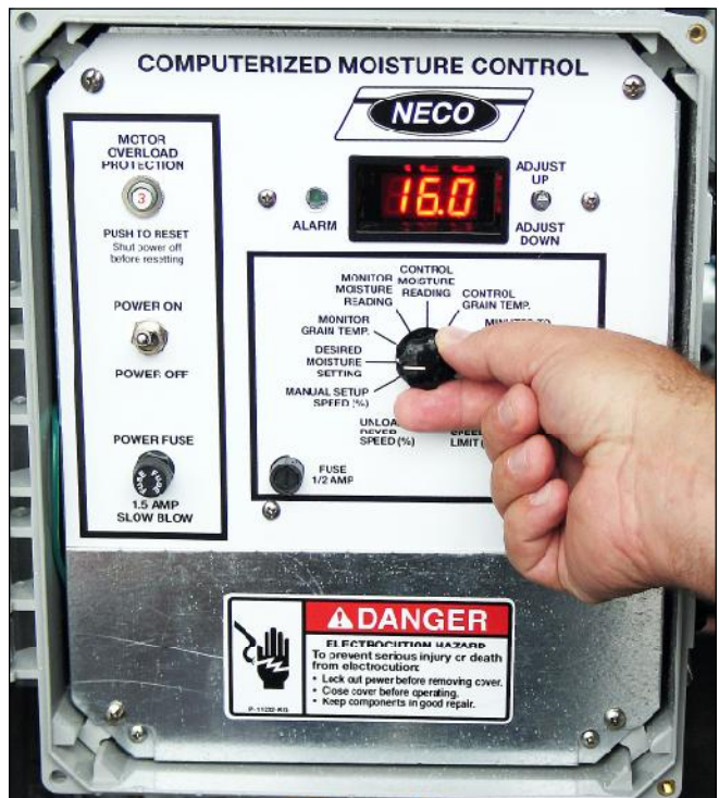
Figure 5.3 - Set the Desired Moisture Setting
